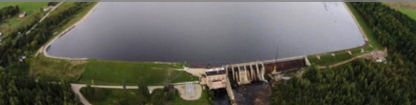
UPPCO Boney Falls Hydroelectric Dam
